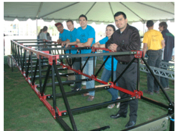
Student team has assembled the steel bridge in preparation for the competition.
